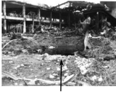
MEK Peroxide Storage Tank Explosion (exposed to external fire)
